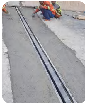
Waterproof of building expansion joint
