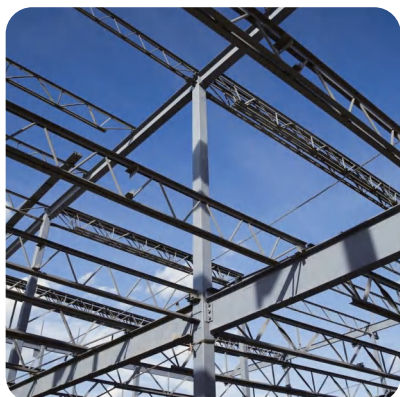
Steel structure seal
