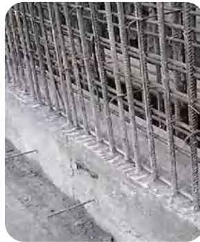
Structure construction waterproof
