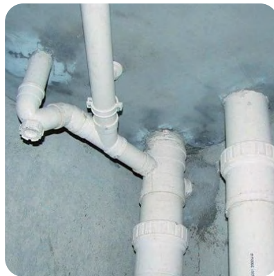
House waterproof seal
