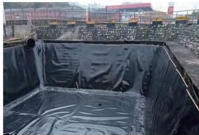
Fish pond impermeable membrane bonding
