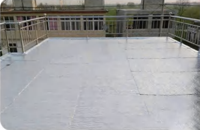
Outdoor balcony construction
